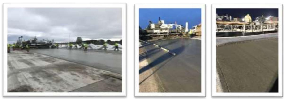
In-Pavement Lights – Can Installation and Setting Can Elevation
