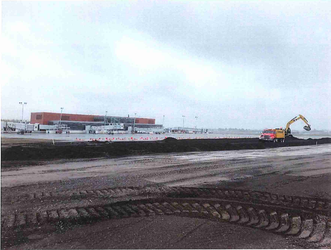
Batch plant preparation:
