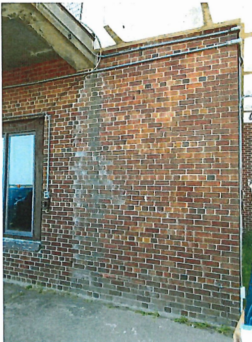
Photo 2 Cracks in brick masonry and mortar joints in need of tuck-pointing
