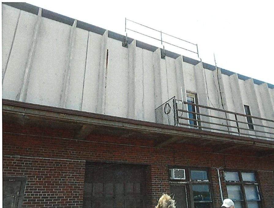
Photo 3 Upper precast concrete wall panels paint finish peeling
