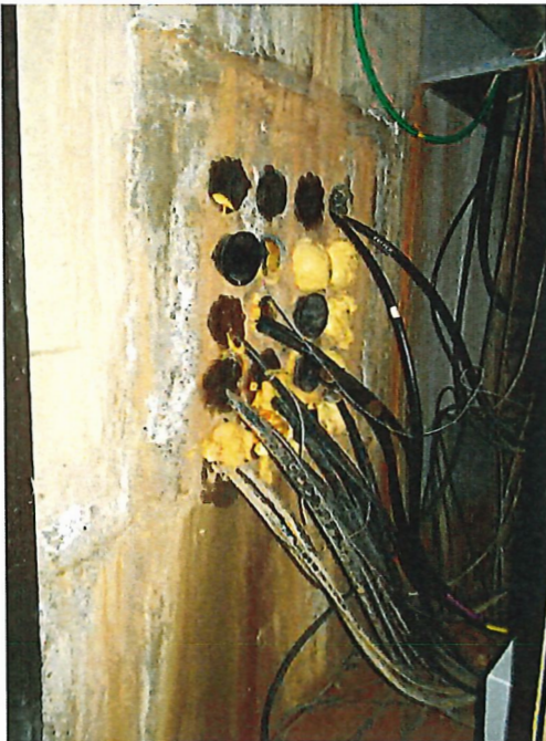
Photo 5 Water Intrusion coming in along pipe/ conduit penetrations in lower mechanical room
