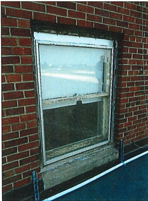
Photo 8 Exterior painted wood framed windows in need of replacement
