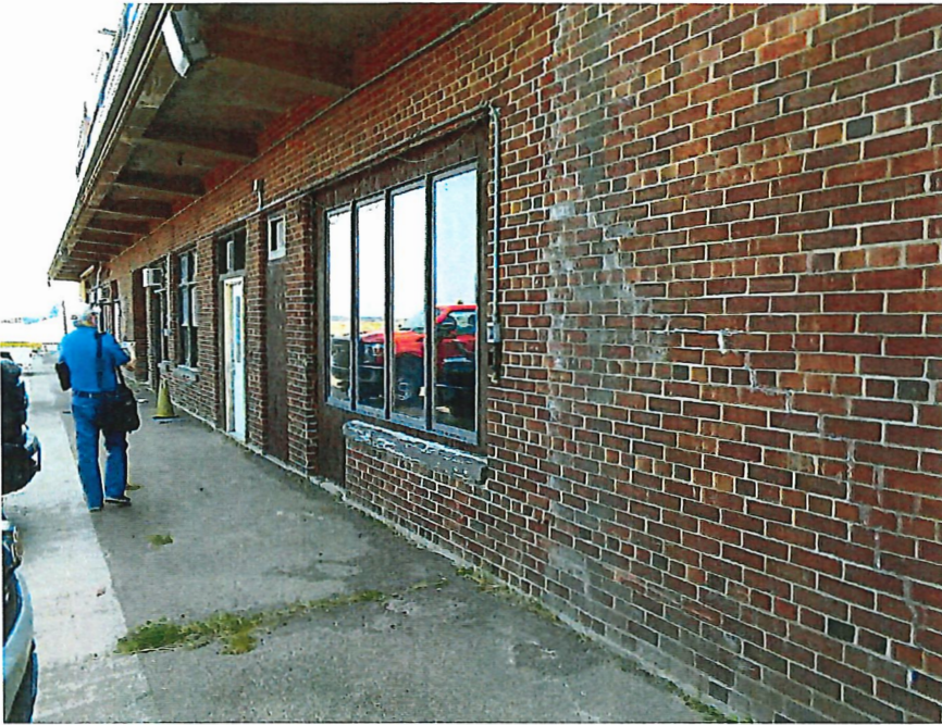
Photo 4 Infilled openings along North wall had no flashing or sealant present
