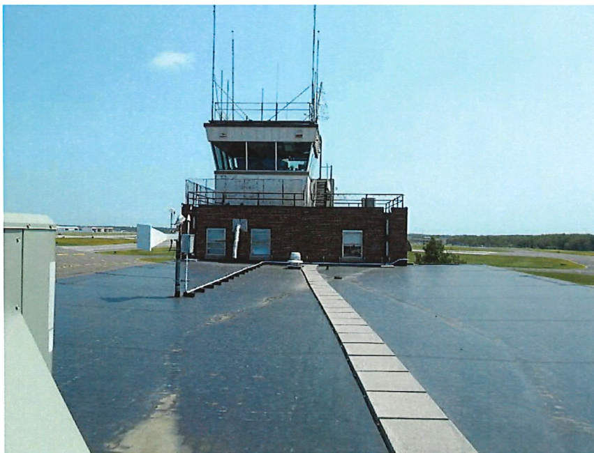
Photo 10 EPDM single-ply roof membrane
