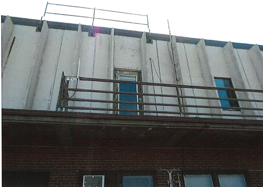
Photo 9 Exterior painted wood door and frame in need of replacement
