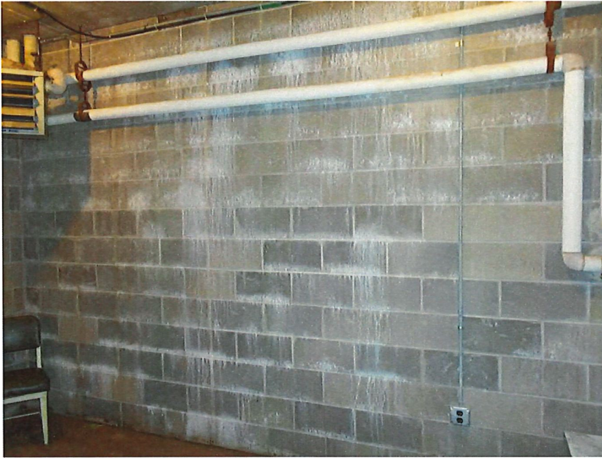
Photo 6 Efflorescence on masonry (CMU) wall in mechanical room
