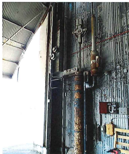
Photo 4 Hydraulic System That Operates Hangar Doors
