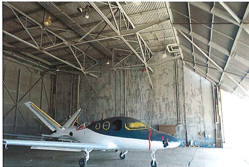
Photo 2 Peeling Paint at Interior Metal Liner Panel
