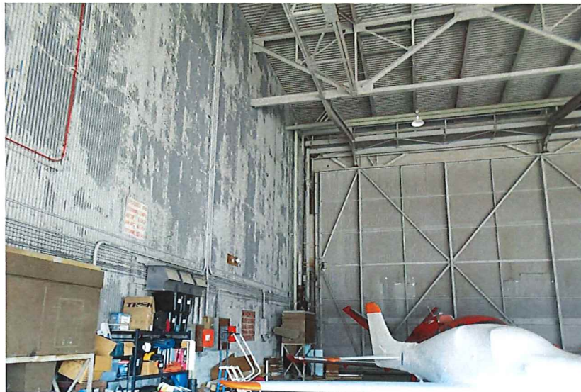
Photo 3 Damage at North Side Hangar Door / Peeling Paint at Interior Metal Liner Panel
