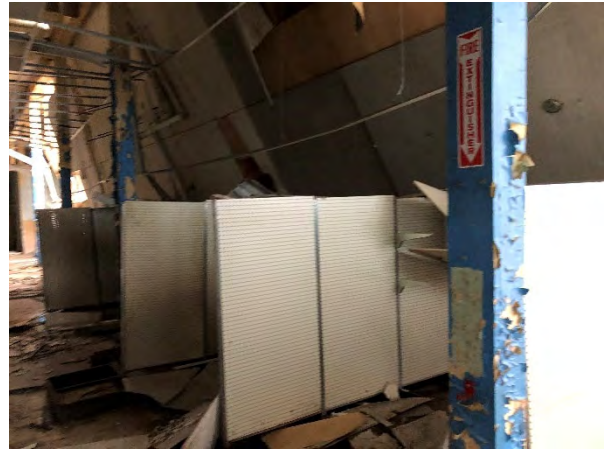
Photo 50 Storage (Room #15) entire south wall collapsed
