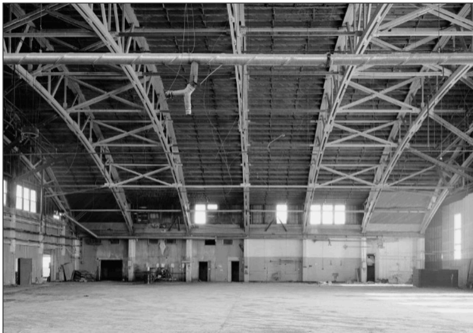
Figure 6. Ellsworth Readiness Hangar, Interior Wooden Crescent Arched Trusses (McCormick and Hufstetler 1994)
