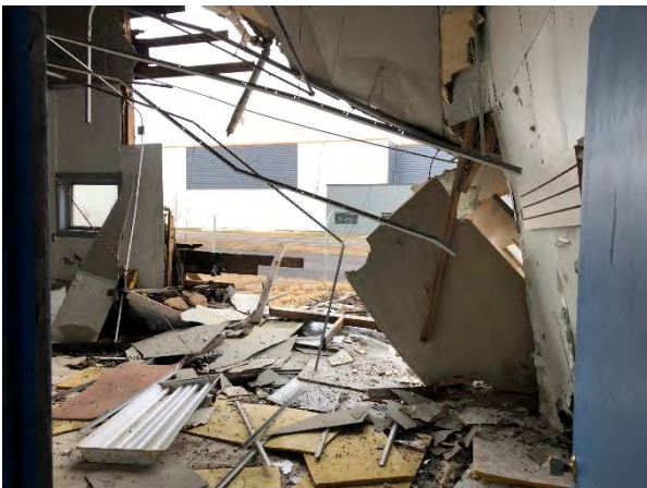
Photo 53 Storage (Room #16) partial south wall collapsed
