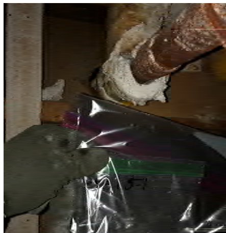
Photo 10 Room #20 2 nd floor pipe wrap (23% Amosite 6% Chrysotile)
