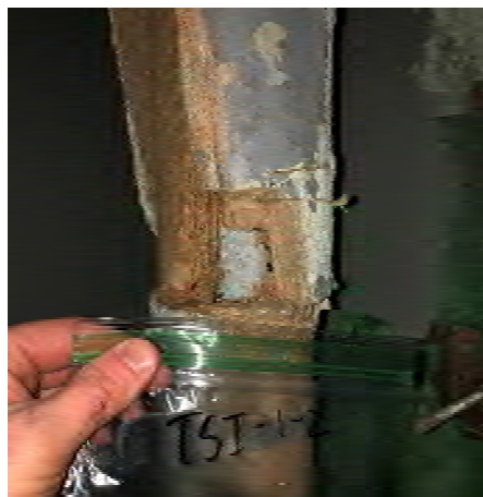
Photo 8 Stock room C white pipe wrap (3% Chrysotile) and Brown pipe wrap (56% Chrysotile)
