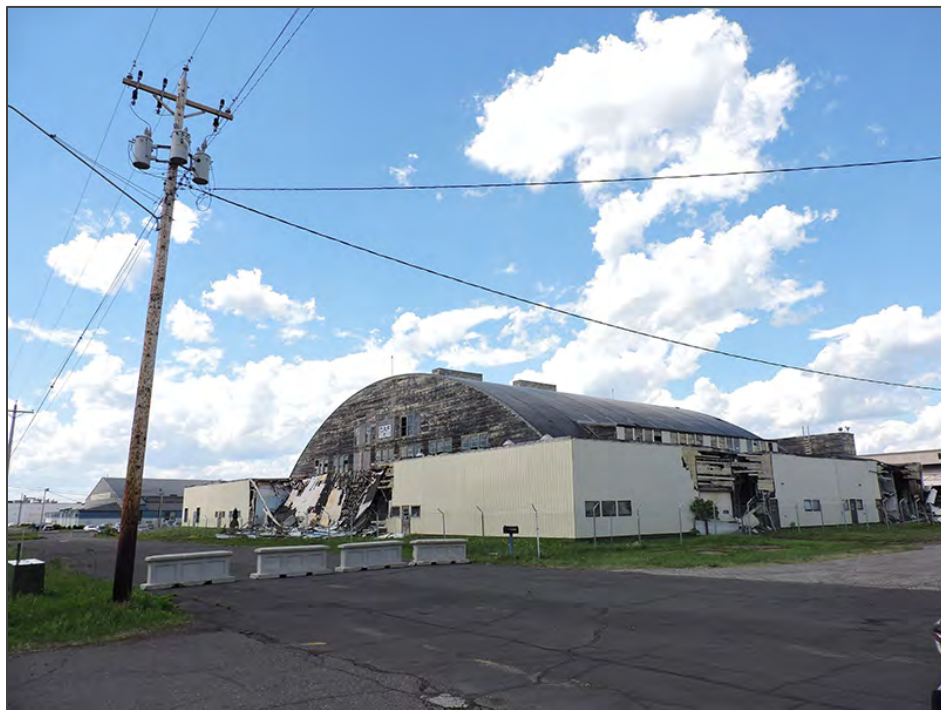
Figure 3. Hangar 101, Facing Northwest, Showing Collapsing Wings (106 Group, May 2021)
