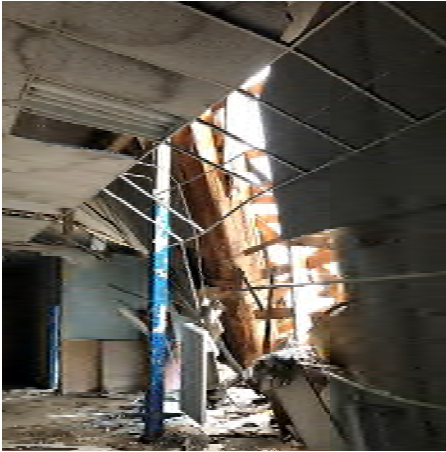
Photo 51 Storage (Room #15) entire south wall collapsed
