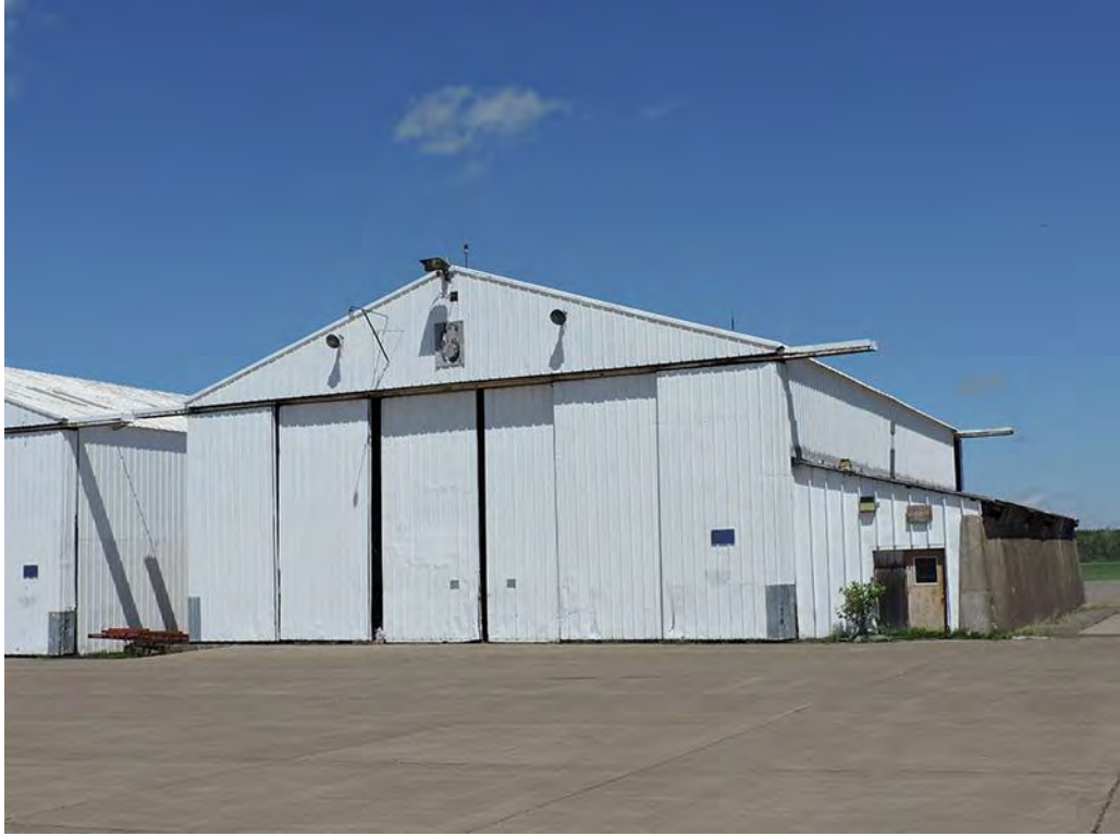
SL-DUL-3644 - 5/25/2021 - South Elevation, Facing North-Northwest
