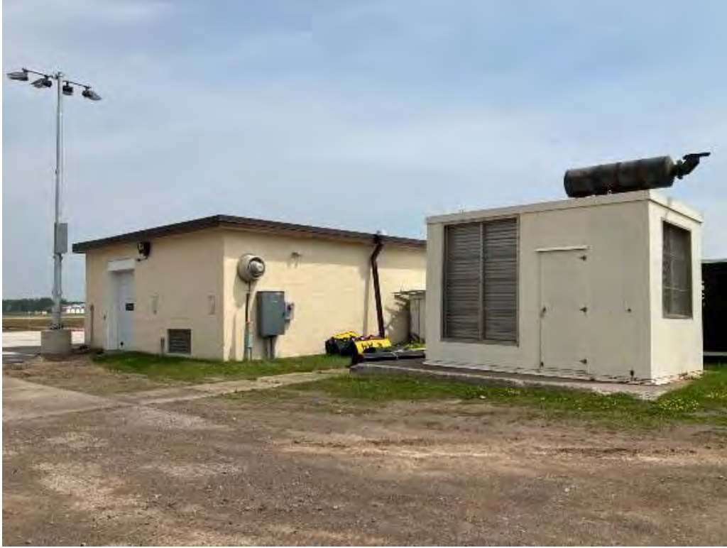
SL-DUL-4033 - 7/25/2023 - Building 301, West-Facing Façade, South Elevation, and Mechanicals Outbuilding, Facing Northeast
