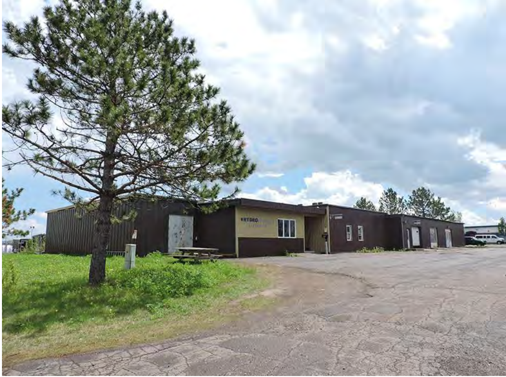
SL-DUL-3646 - 5/25/2021 - North & West Elevations, Facing Southeast
