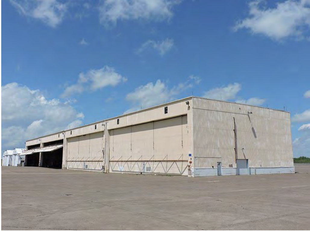
SL-DUL-3645 - 5/25/2021 - South & East Elevations, Facing Northwest
