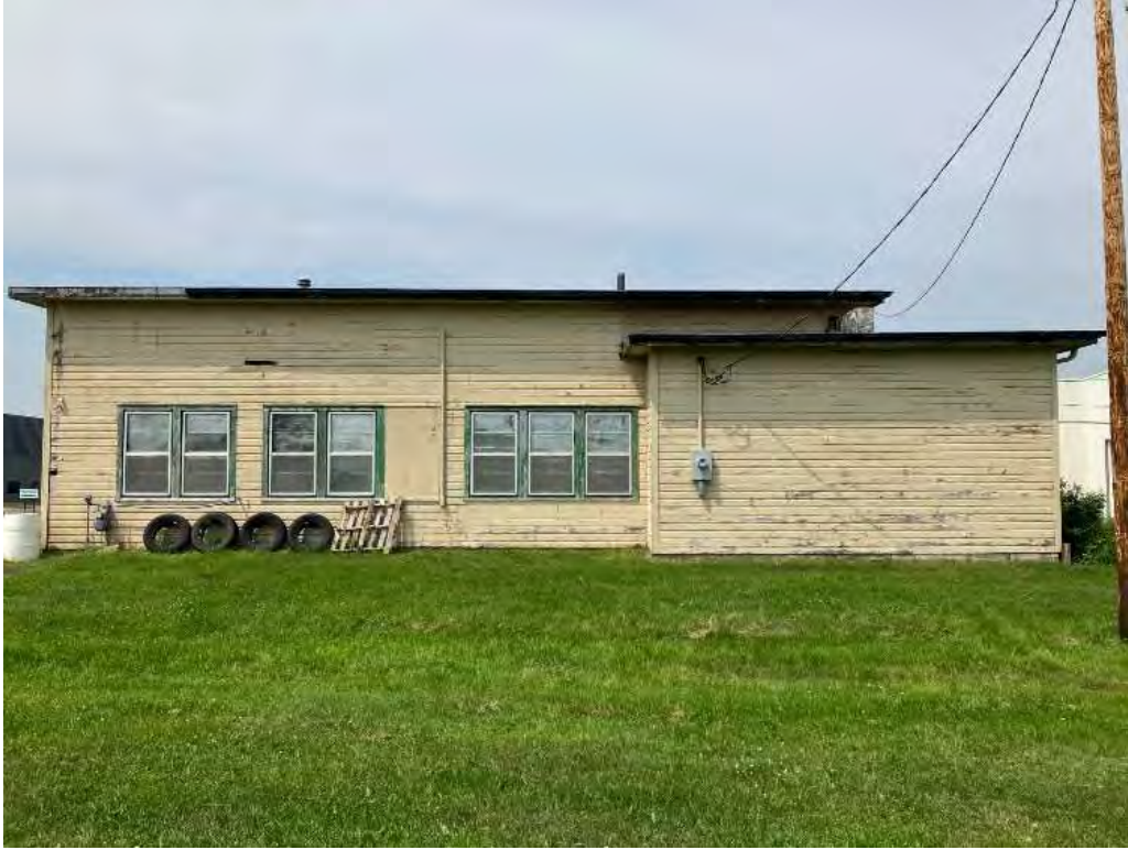
SL-HER-040 - 7/25/2023 - East Elevation, Facing West
