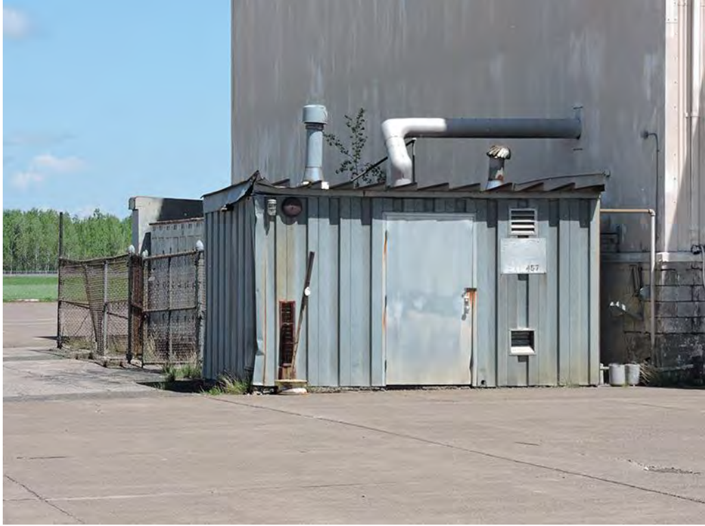
SL-DUL-3645 - 5/25/2021 - Structures on West Elevation, Facing Northeast
