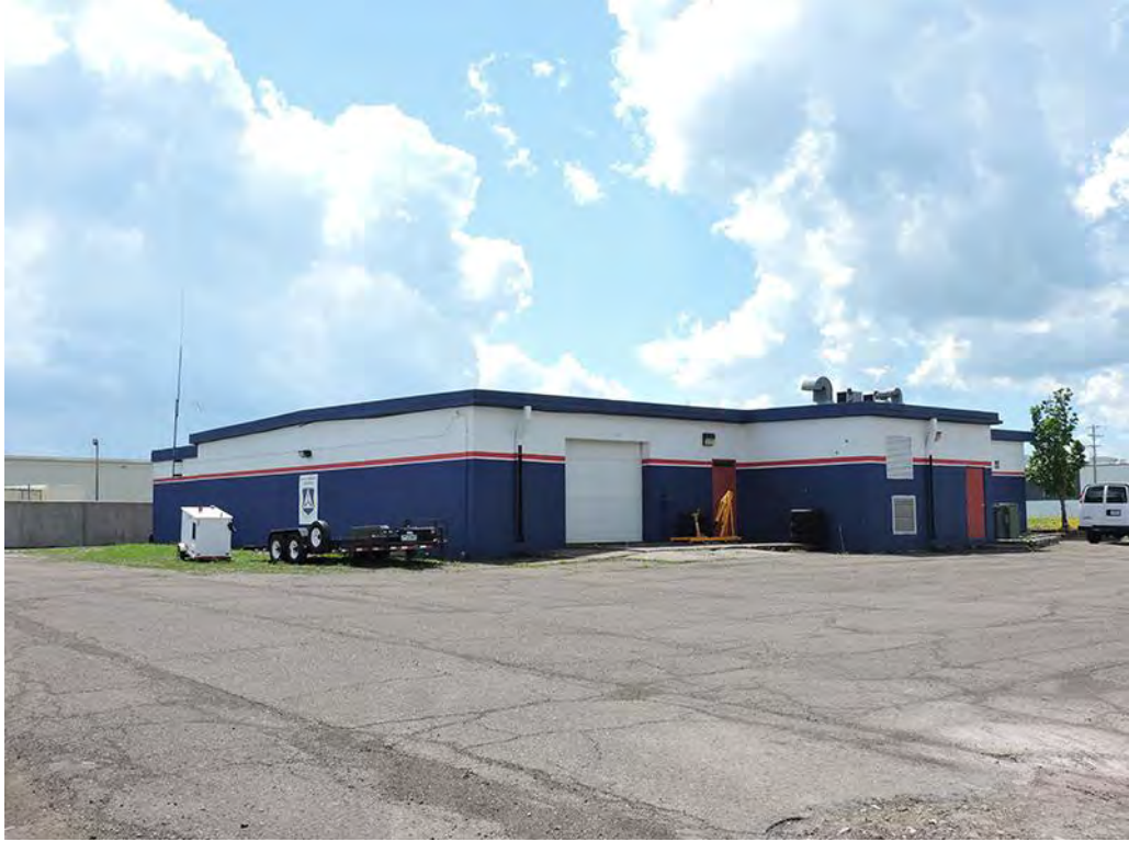
SL-DUL-3647 - 5/25/2021 - North & West Elevations, Facing Southwest
