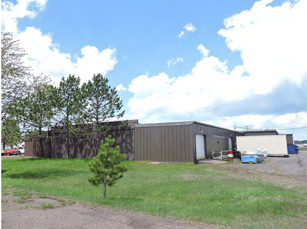
SL-DUL-3646 - 5/25/2021 - South & East Elevations, Facing Northwest
