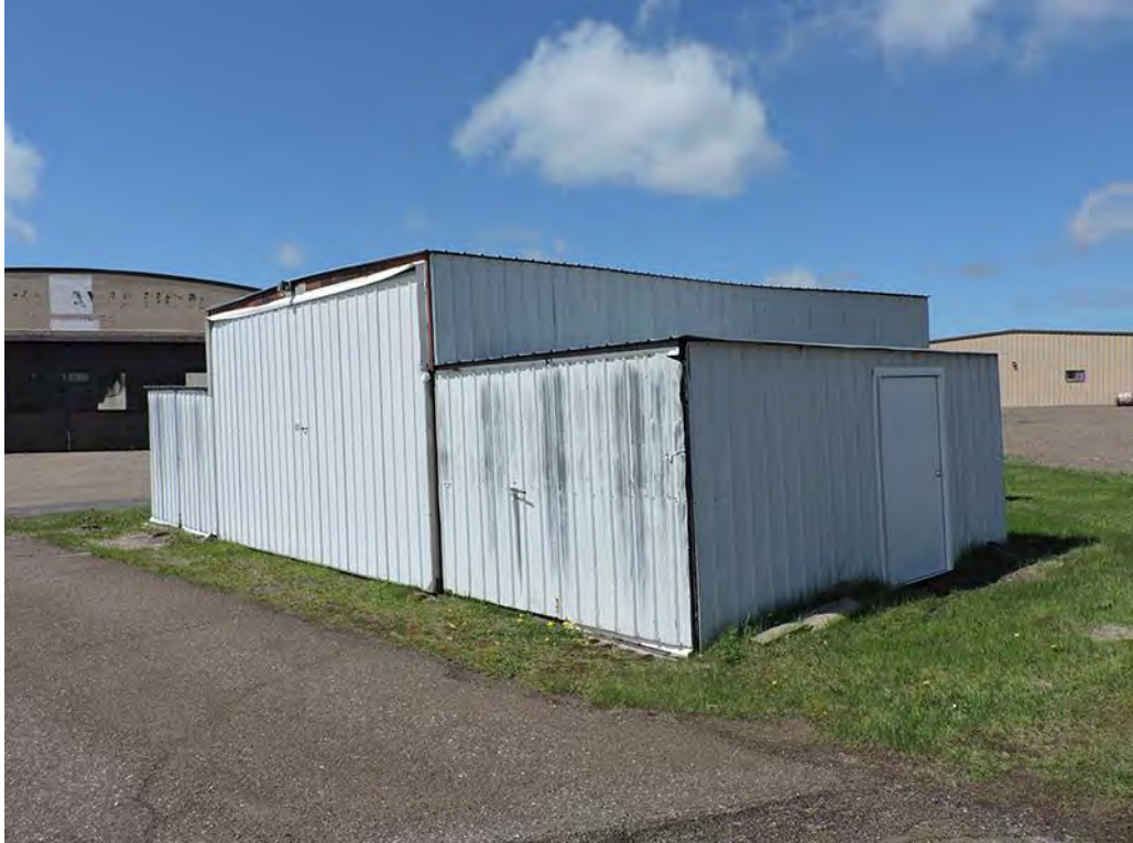
SL-DUL-3637 - 5/25/2021 - East & North Elevations, Facing Southwest
