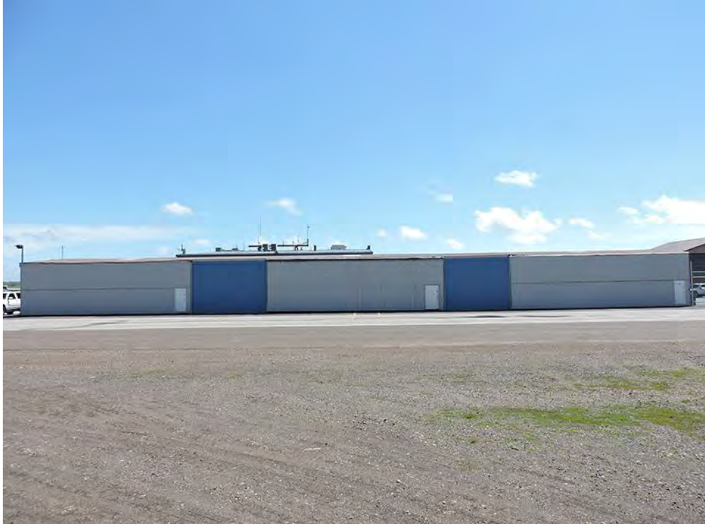
SL-DUL-3639 - 5/25/2021 - West Elevation, Facing East
