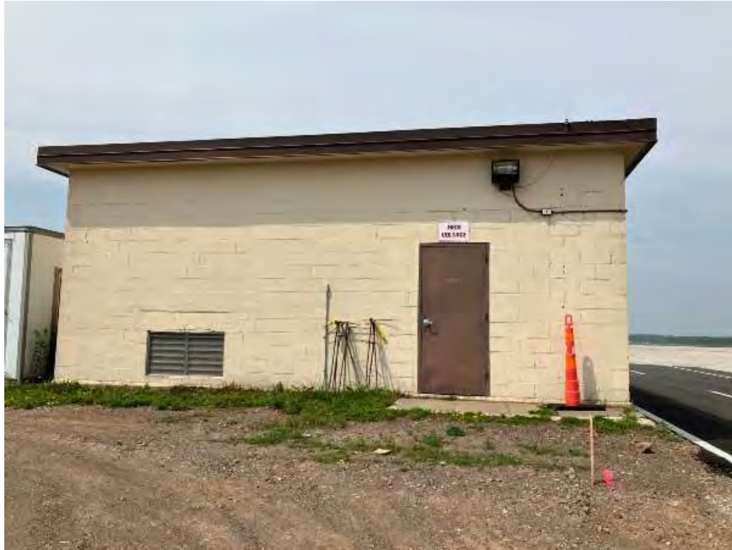
SL-DUL-4033 - 7/25/2023 - Building 301, East Elevation, Facing West
