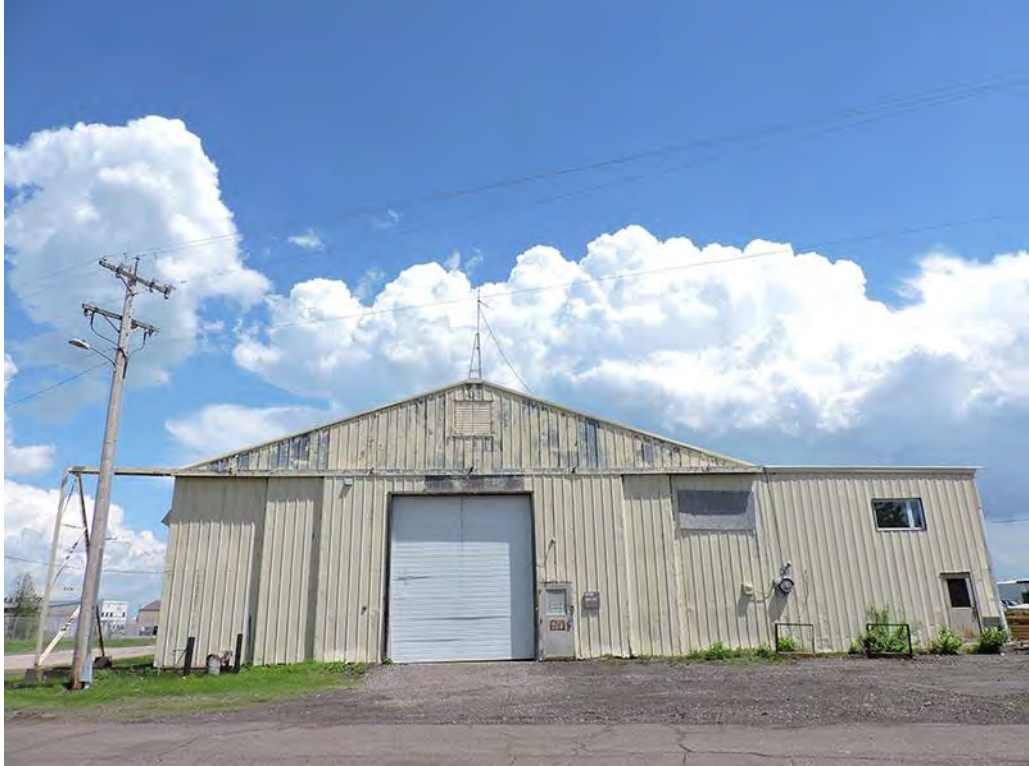
SL-DUL-3640 - 5/25/2021 - East Elevation, Facing West
