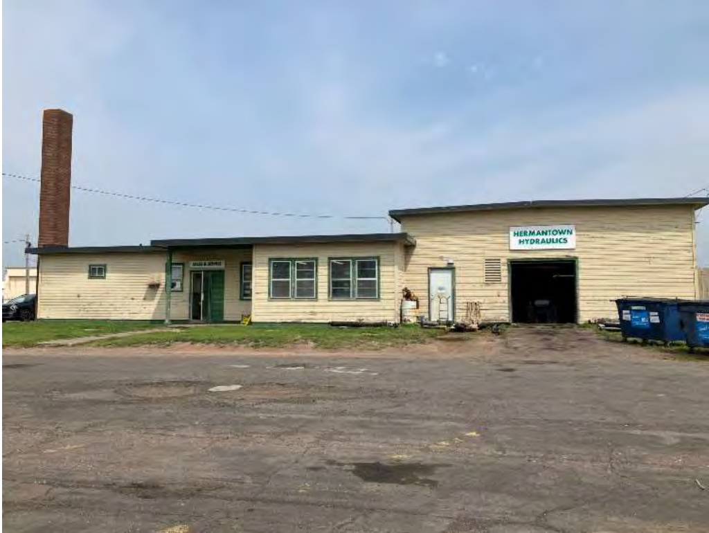
SL-HER-040 - 7/25/2023 - South-Facing Façade, Facing North
