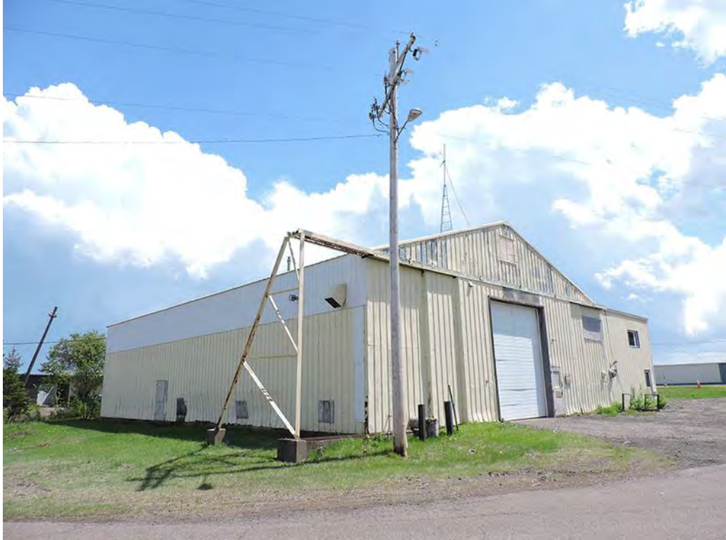
SL-DUL-3640 - 5/25/2021 - East & North Elevations, Facing Northeast
