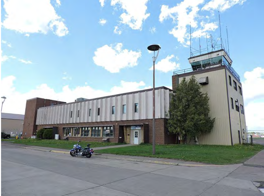
SL-DUL-3638 - 5/25/2021 - West Elevation & Control Tower, Facing Northwest
