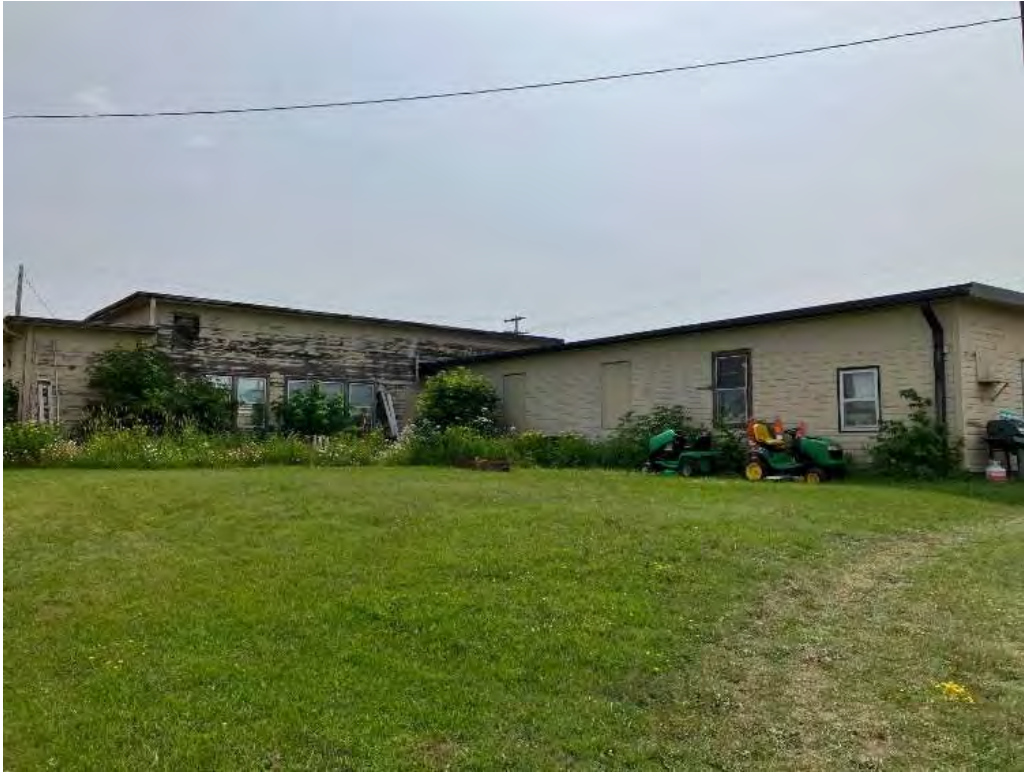
SL-HER-040 - 7/25/2023 - North and West Elevations, Facing Southeast
