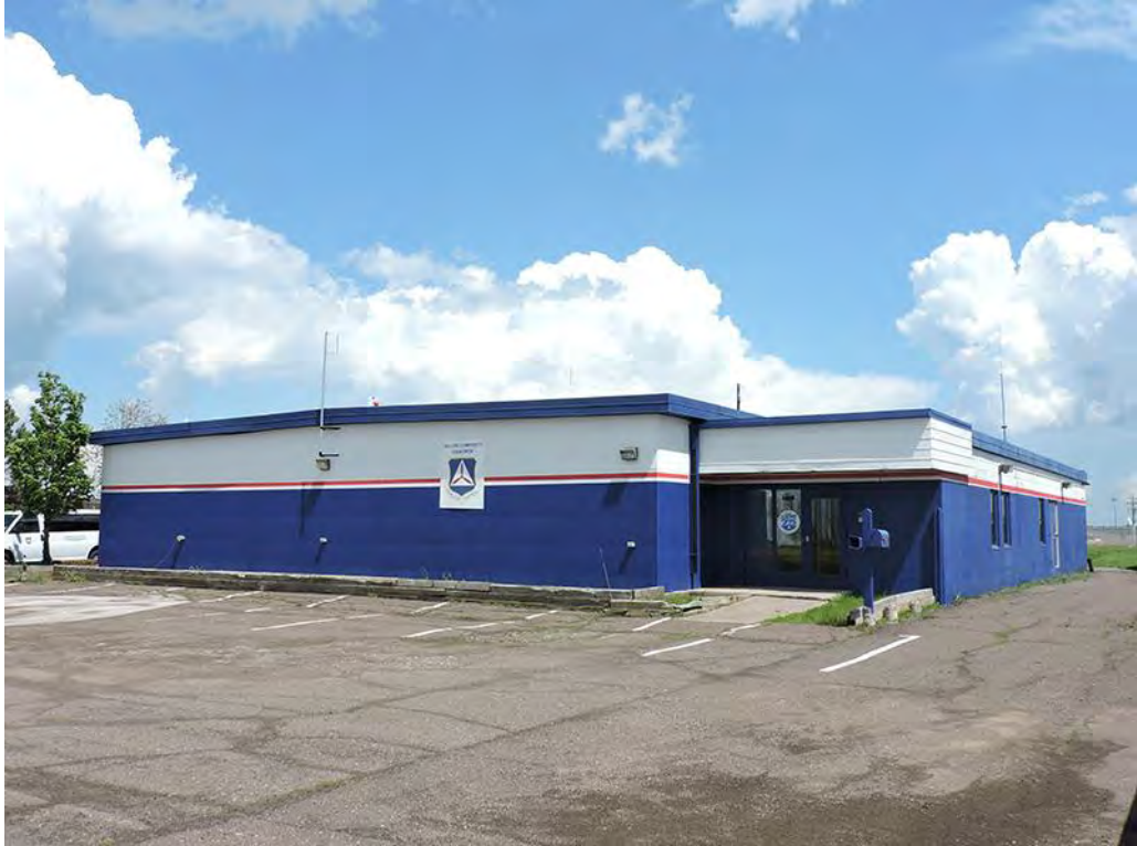
SL-DUL-3647 - 5/25/2021 - South & East Elevations, Facing Northeast
