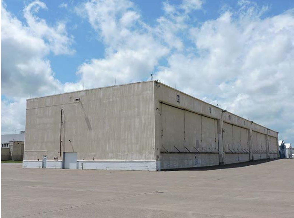
SL-DUL-3645 - 5/25/2021 - East & North Elevations, Facing Southwest
