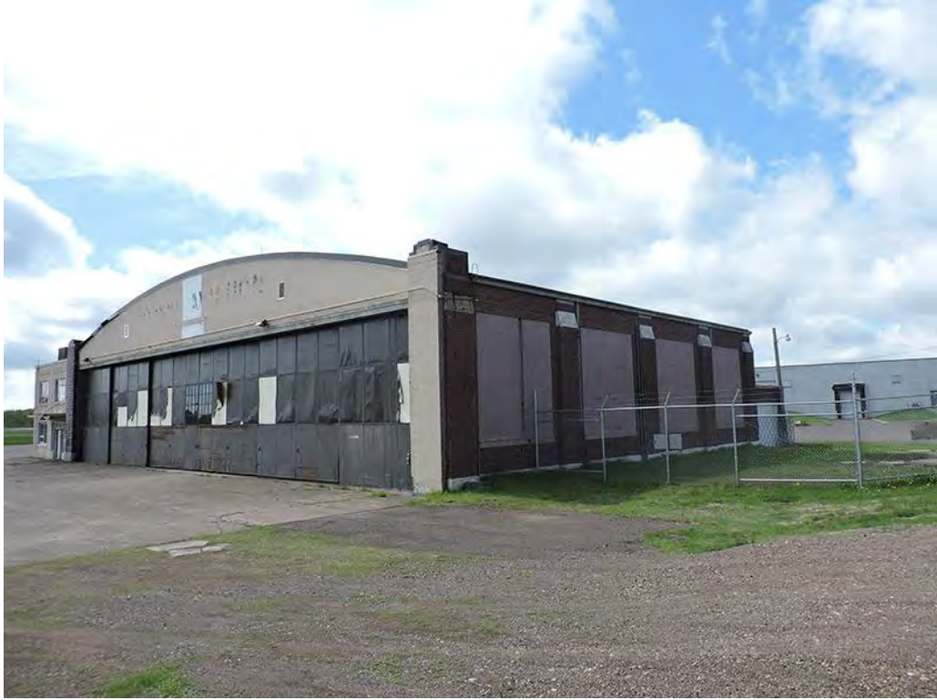
SL-DUL-3636 - 5/25/2021 - Northeast & Southeast Elevations, Facing South
