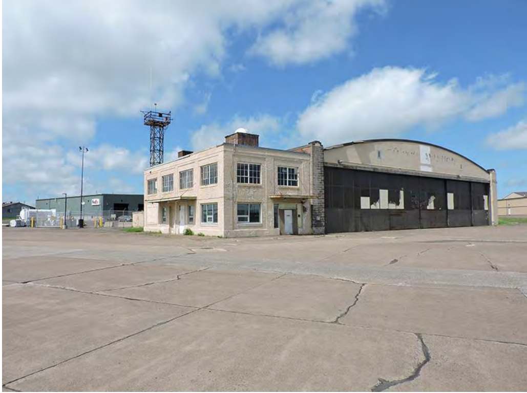
SL-DUL-3636 - 5/25/2021 - Northeast & Northwest Elevations, Facing West-Southwest
