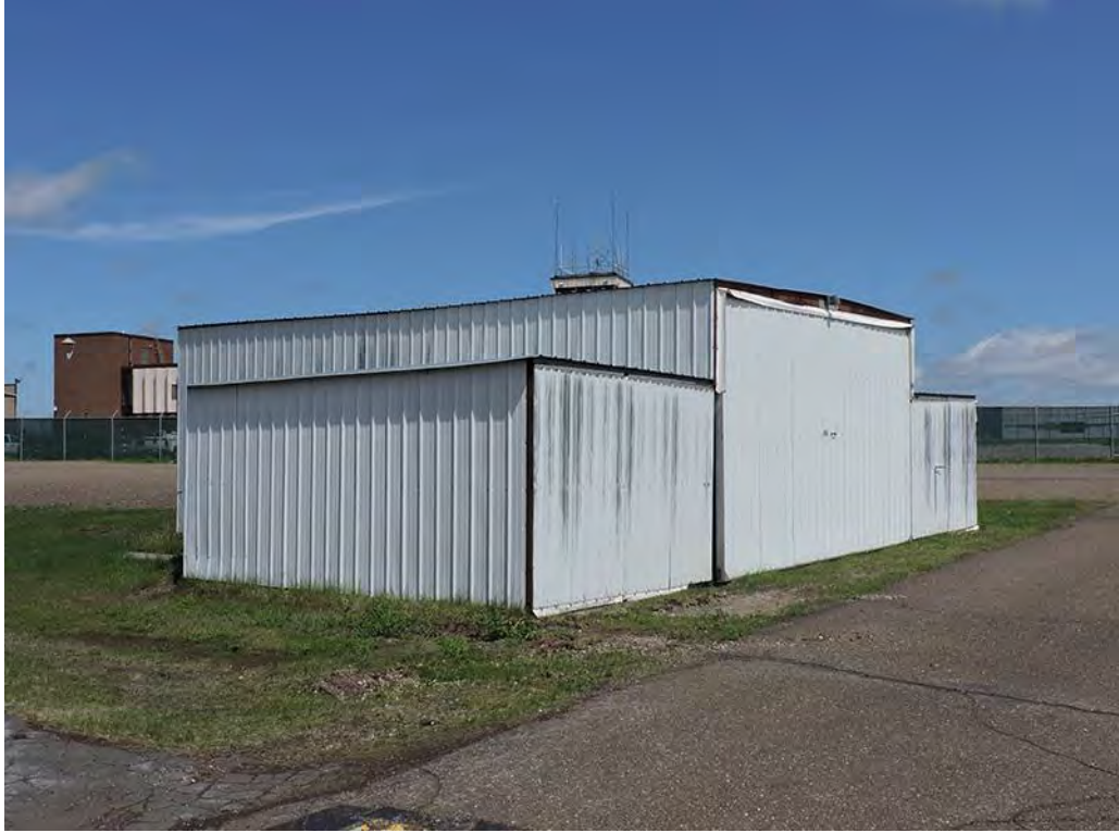
SL-DUL-3637 - 5/25/2021 - East & South Elevations, Facing Northwest
