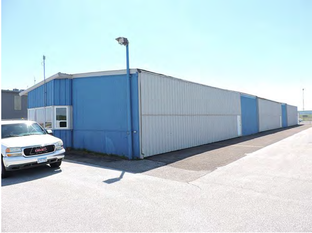
SL-DUL-3639 - 5/25/2021 - North & East Elevations, Facing Southeast
