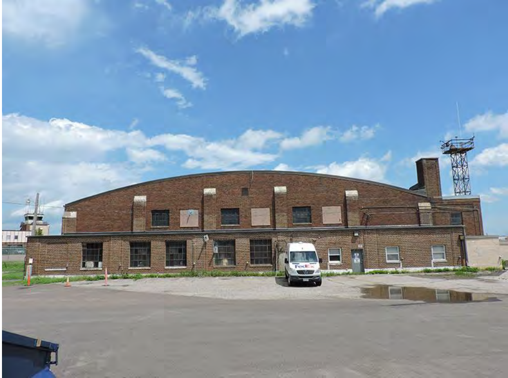
SL-DUL-3636 - 5/25/2021 - Southwest Elevation, Facing Northeast
