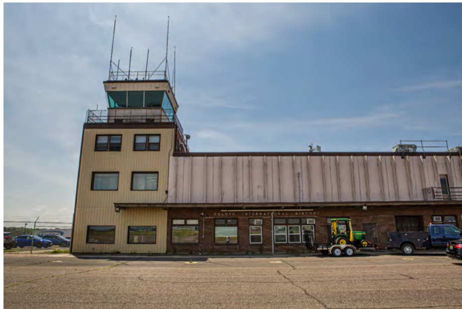
Photo 4 Airside View (from North)
