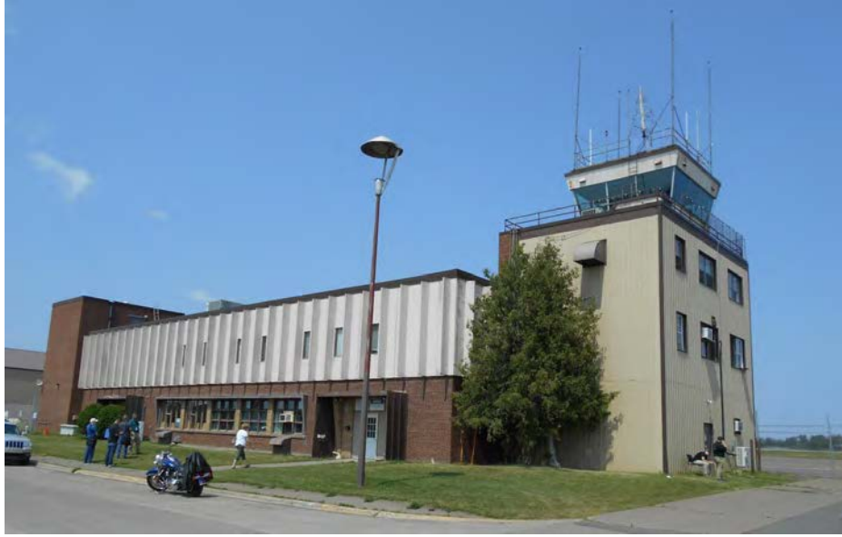
Photo 1 Landside View (from South)
