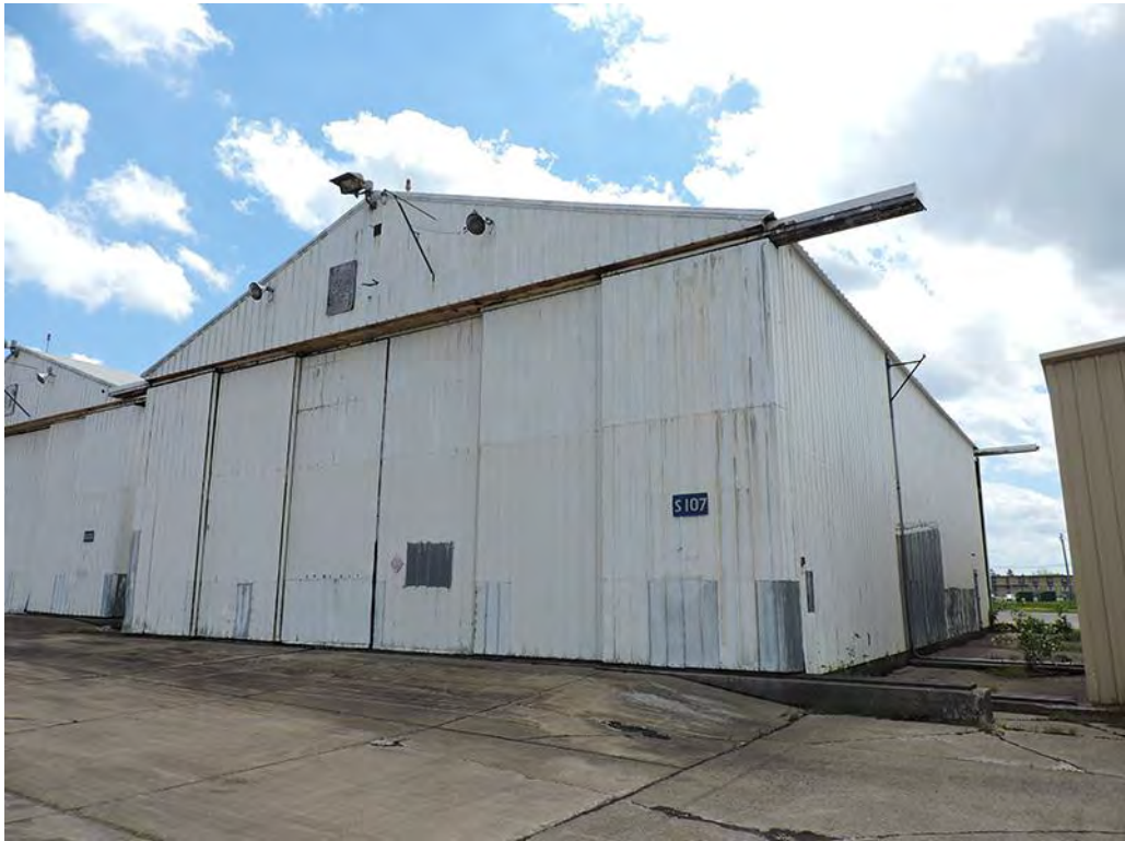
SL-DUL-3642 - 5/25/2021 - North Elevation, Facing Southeast
