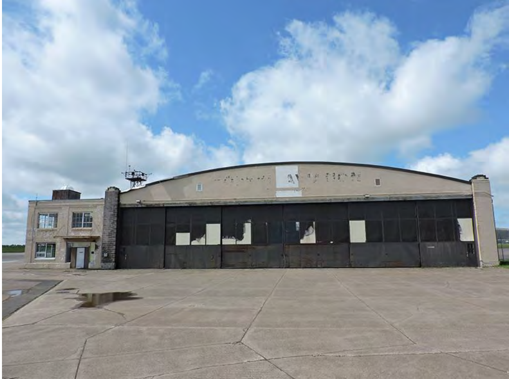
SL-DUL-3636 - 5/25/2021 - Northeast Elevation, Facing Southwest
