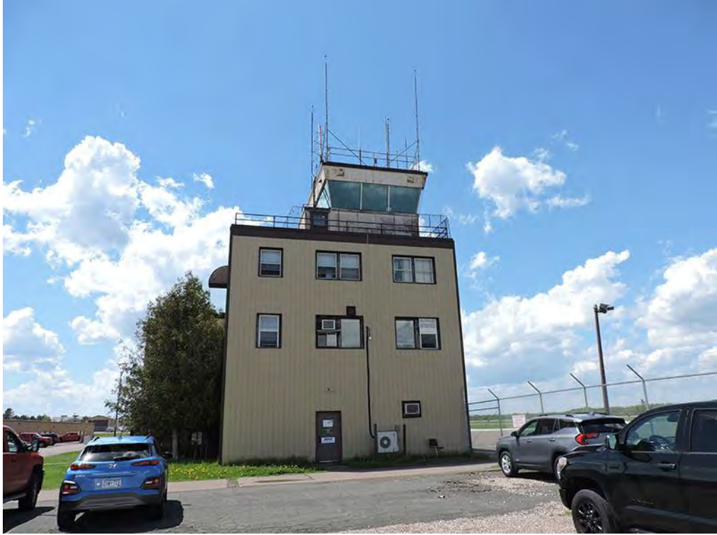
SL-DUL-3638 - 5/25/2021 - East Elevation of Control Tower, Facing South
