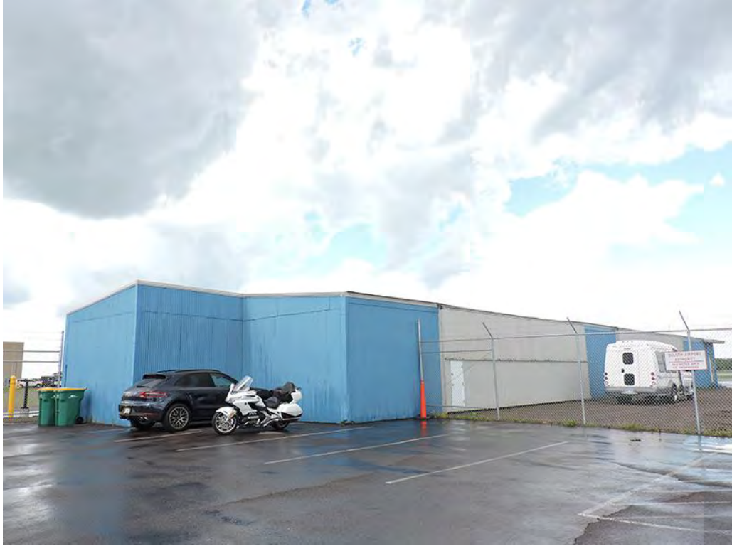
SL-DUL-3639 - 5/25/2021 - South & East Elevations, Facing Northwest
