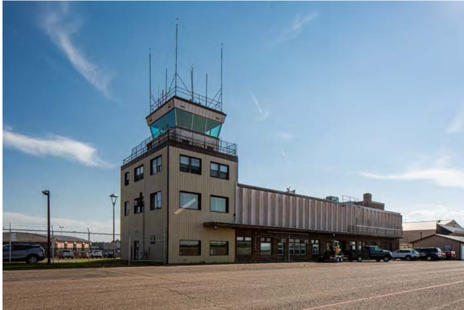
Photo 5 Airside View (from North)
