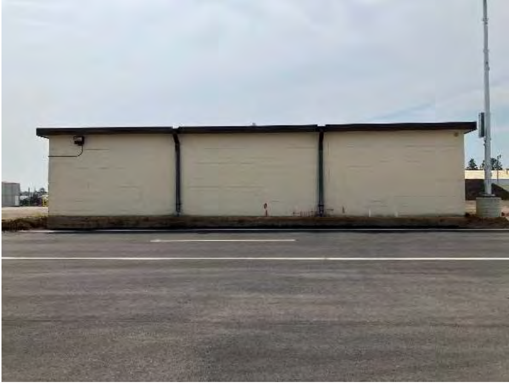
SL-DUL-4033 - 7/25/2023 - Building 301, North Elevation, Facing South
