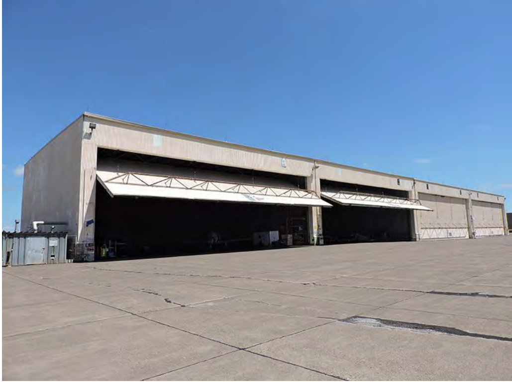
SL-DUL-3645 - 5/25/2021 - South & West Elevations, Facing Northeast
