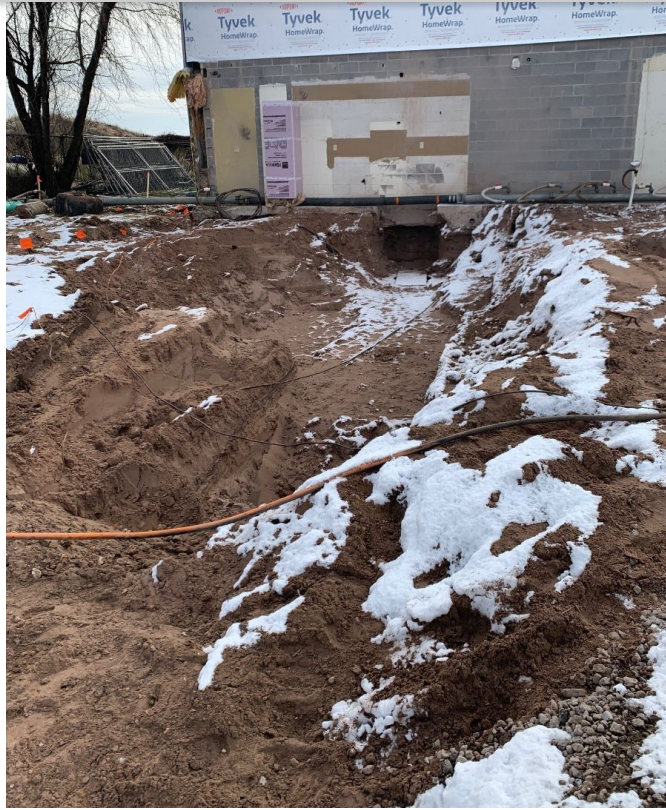
Terminal Building Construction Progress
