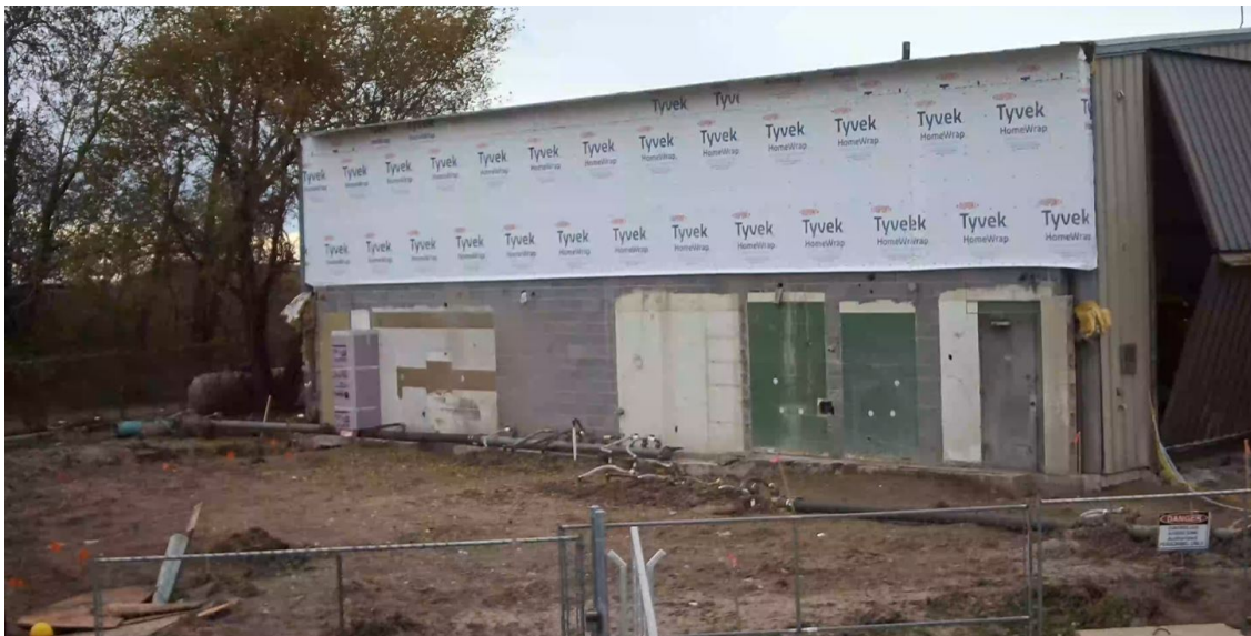
Terminal Building Construction Progress
