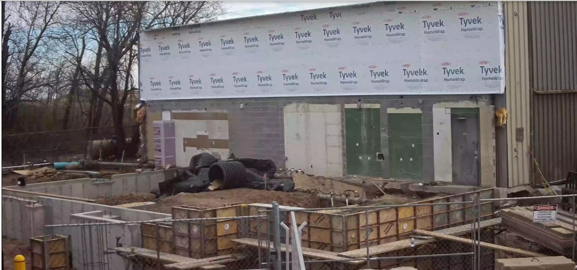
Terminal building construction progress
