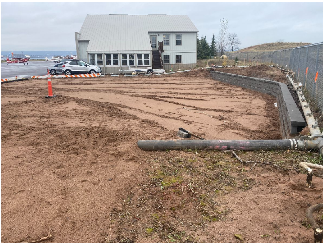
SRE building construction progress
