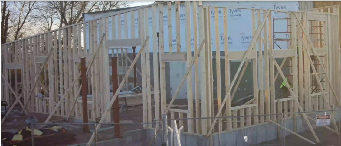
Terminal building construction progress
