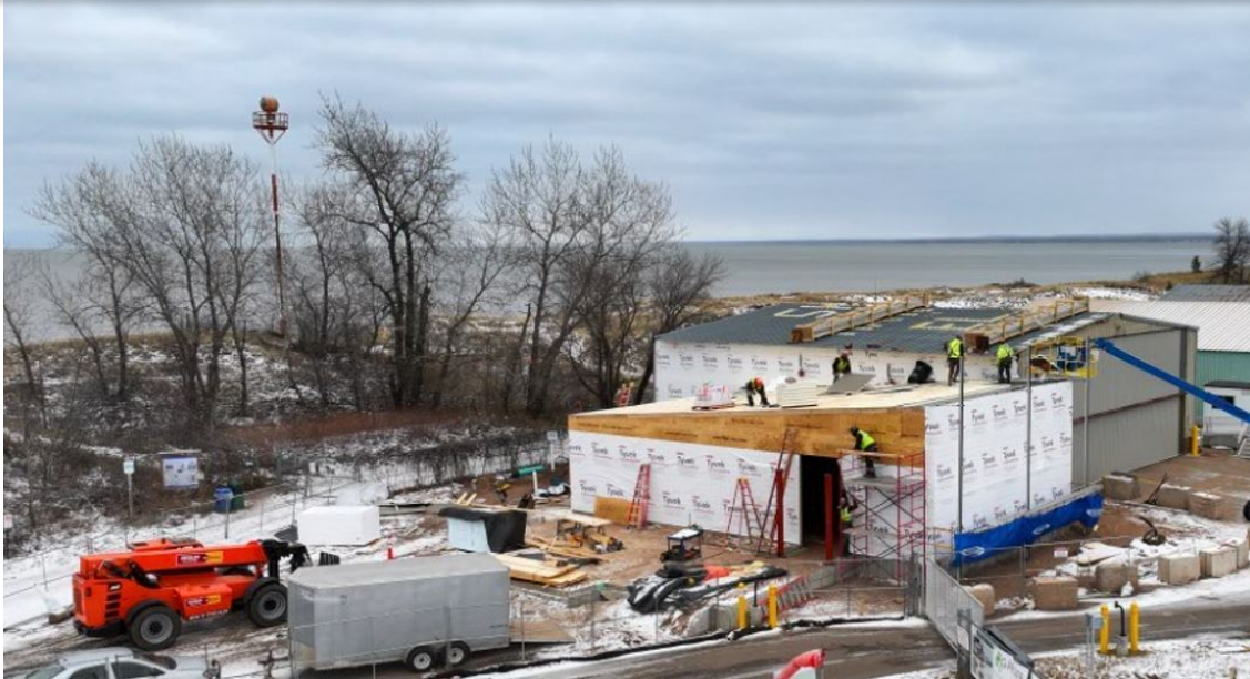
Terminal building construction progress.
