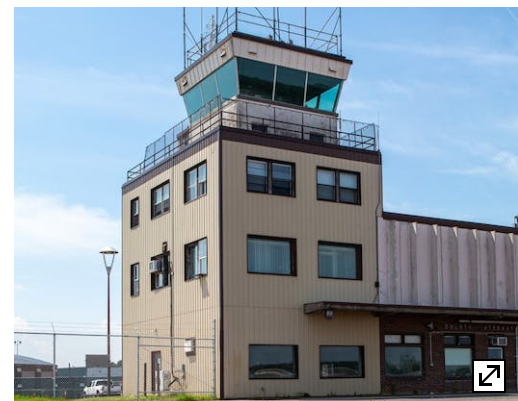
The air traffic control tower at Duluth International Airport.
