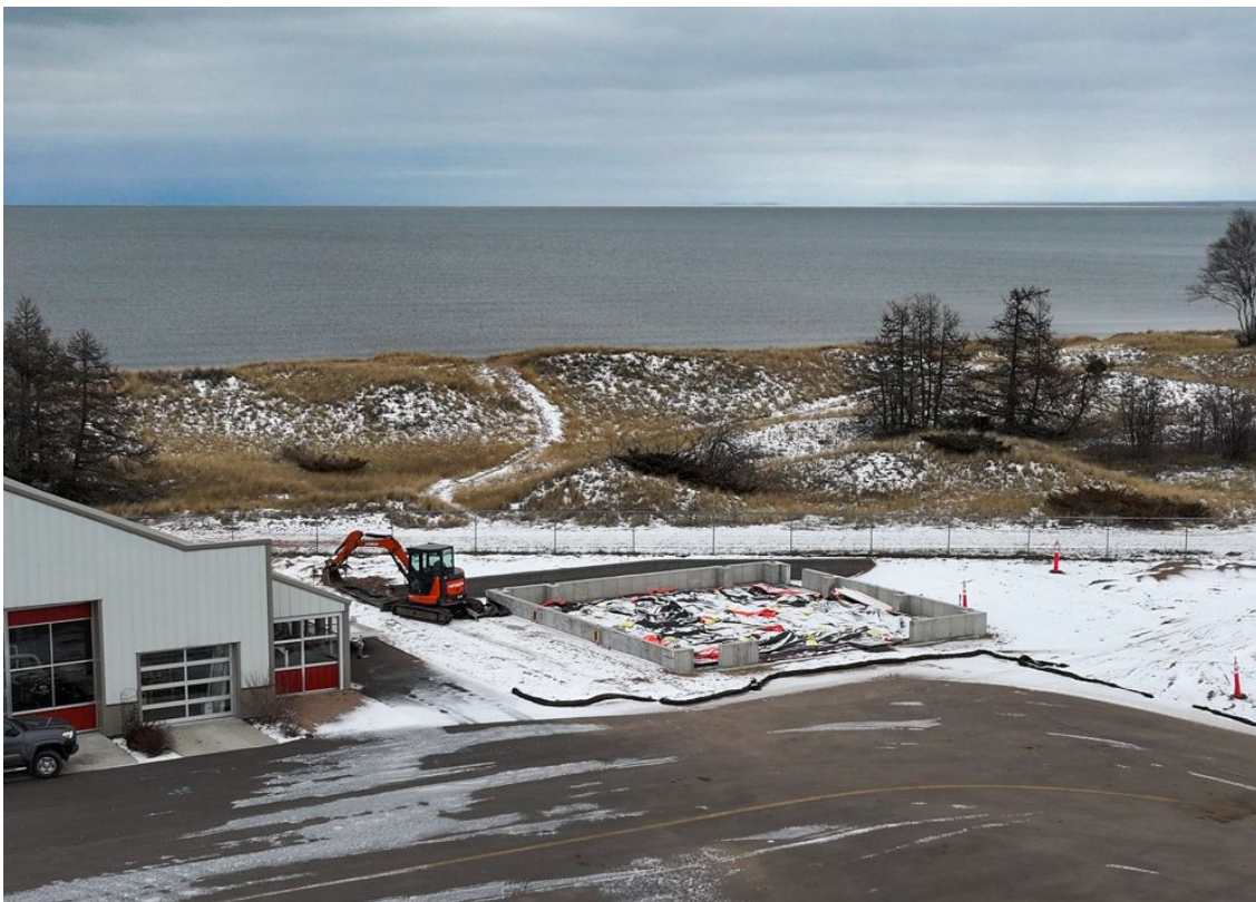
SRE Building construction progress.
