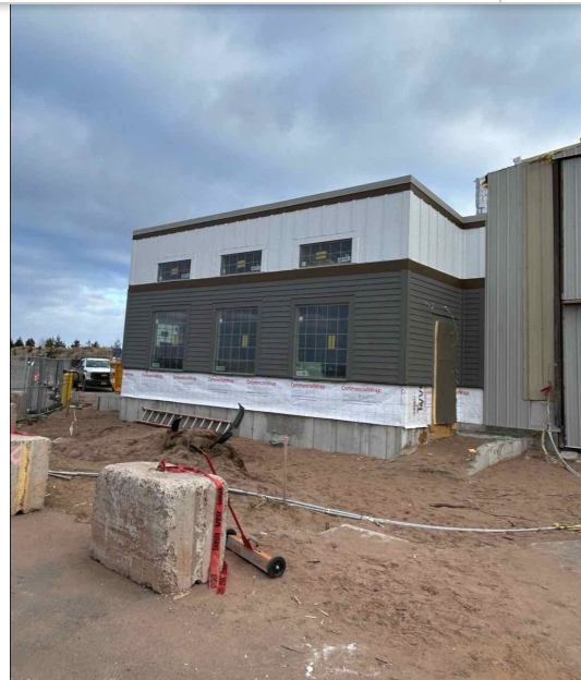
Terminal building construction progress.
