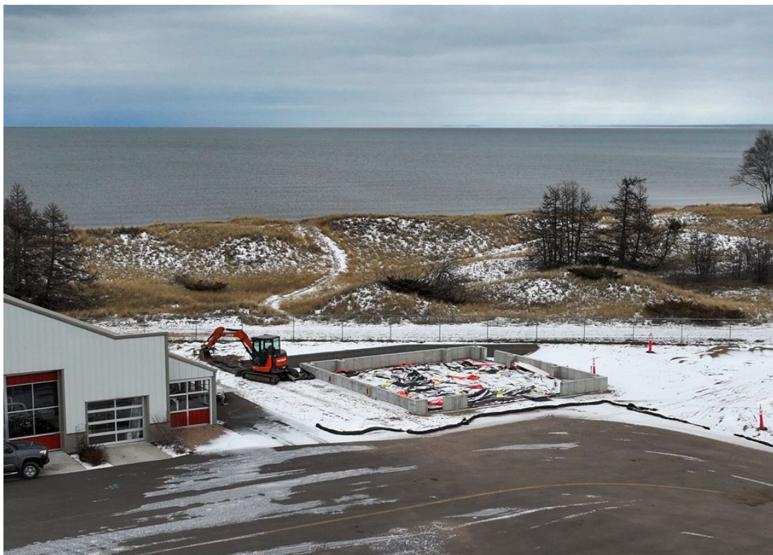
SRE Building construction progress.
