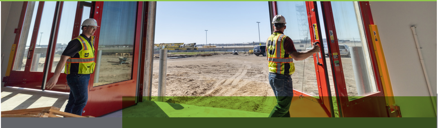
Metropolitan Airports Commission Safety + Security Center, MSP Airport
