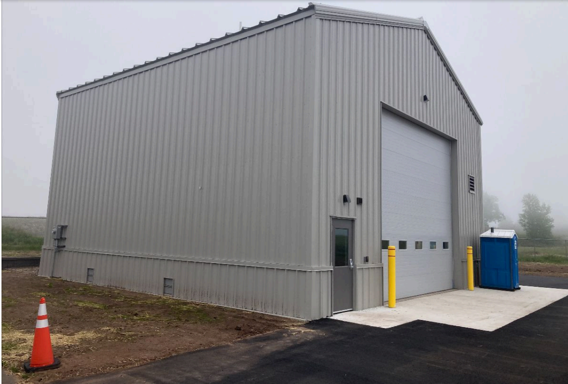
SRE Building construction progress.
