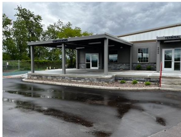
Terminal building construction progress.
