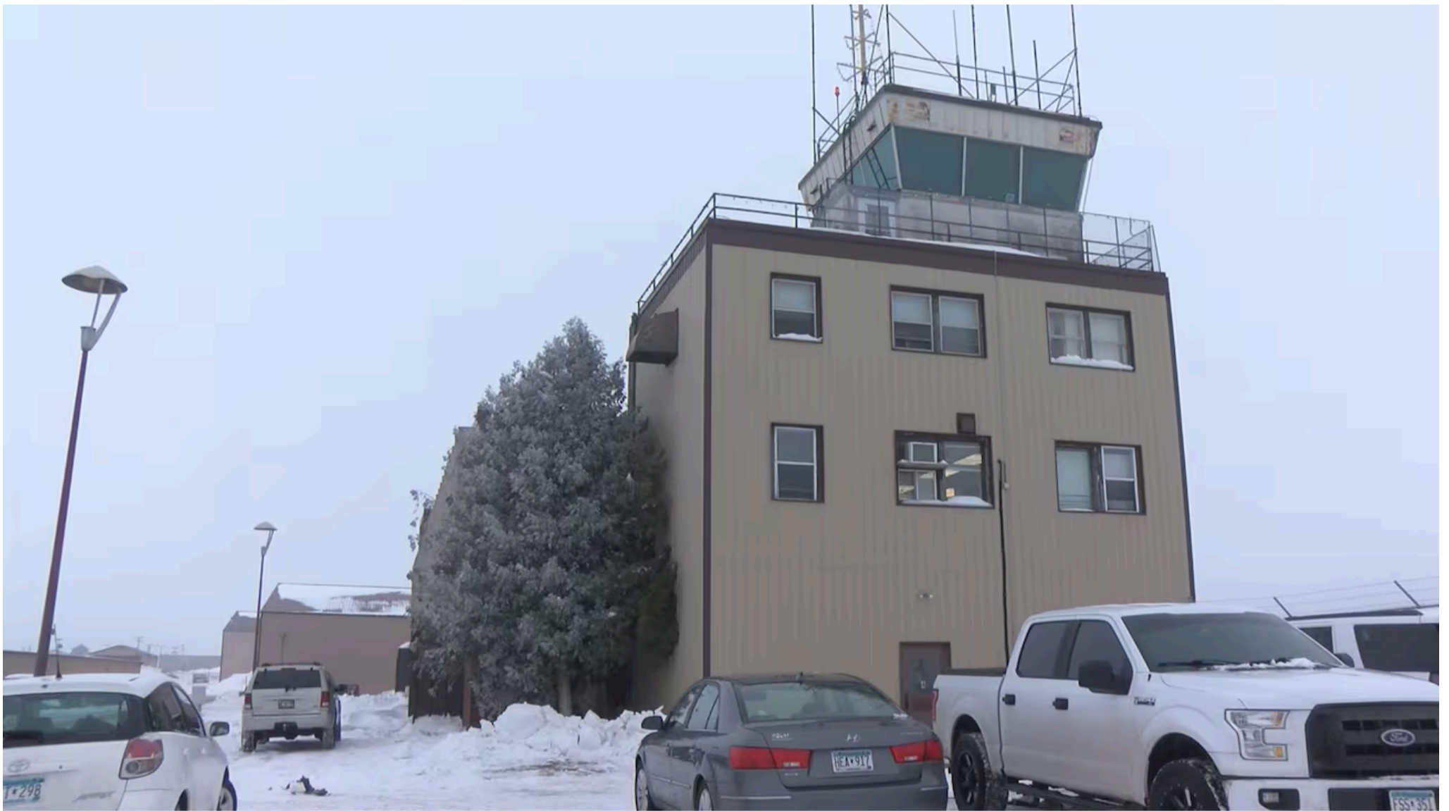
DLH air traffic control tower
