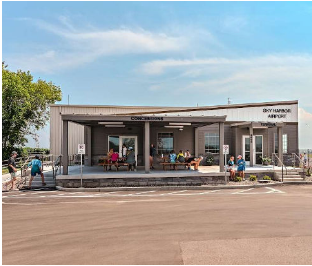
Terminal Building – New Construction in 2024
