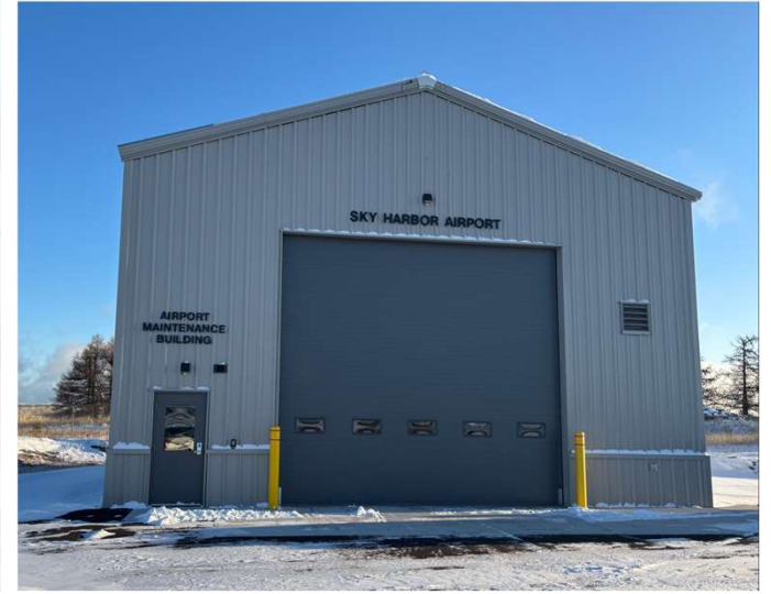
Snow Removal Equipment Building – New Construction in 2024
