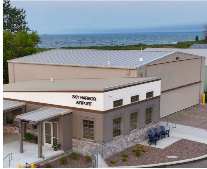
Hangar – Minor Rehabilitation in 2024
